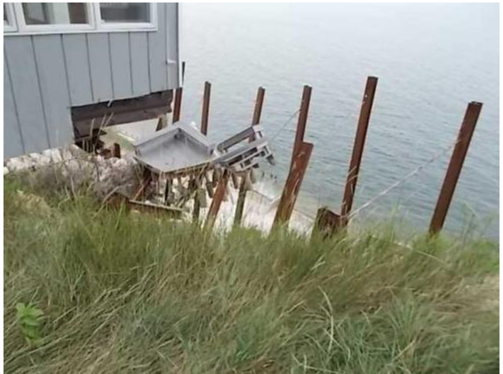
16 Right rear side Date Taken: 7/19/2014 Taken By: Cham Benvenuti Unable to access rear of property due to severe erosion of cliffs
