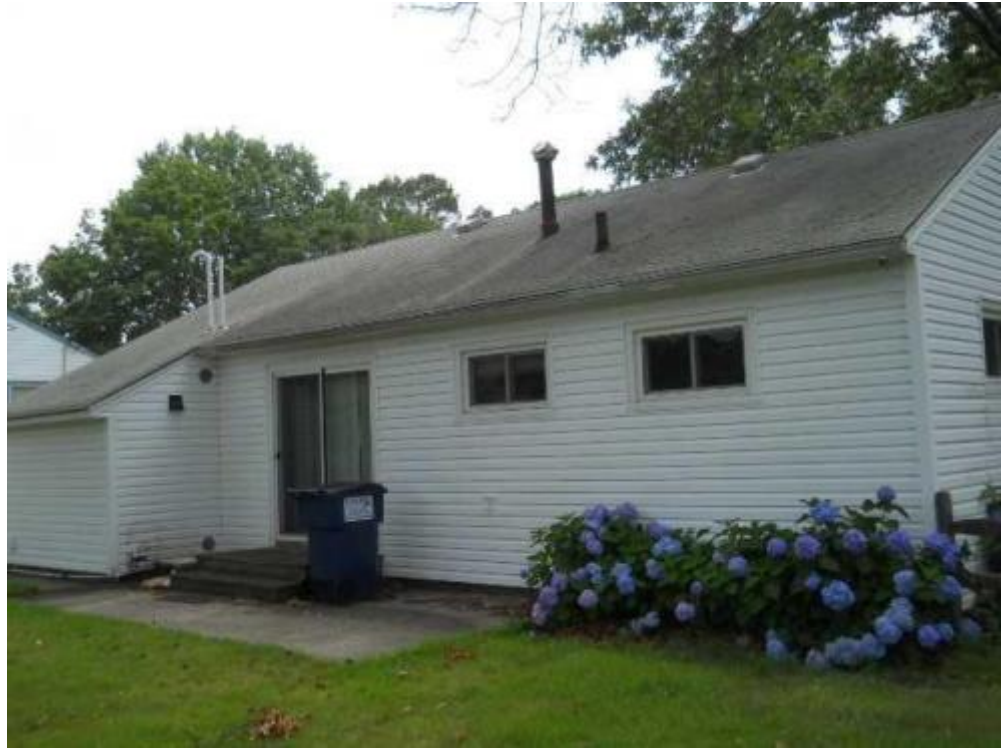
15 rear elevation Date Taken: 7/21/2014 Taken By: Brook Benvenuti
