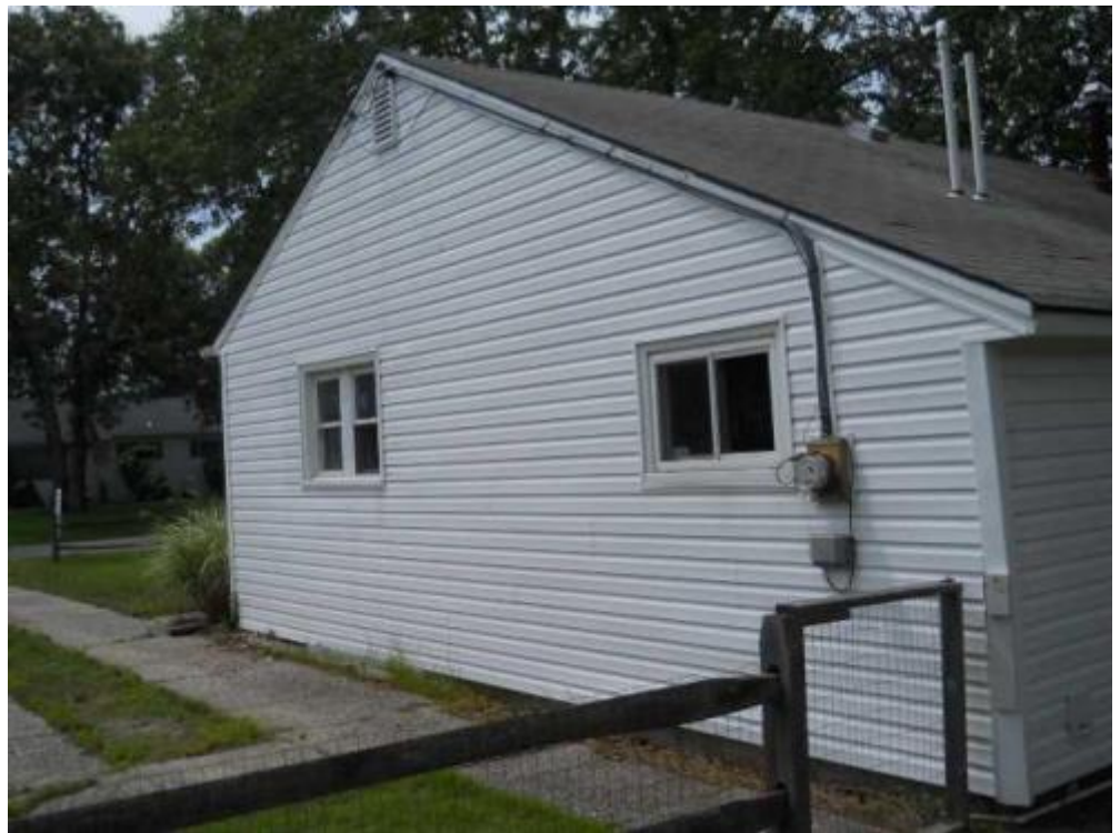
18 right elevation Date Taken: 7/21/2014 Taken By: Brook Benvenuti
