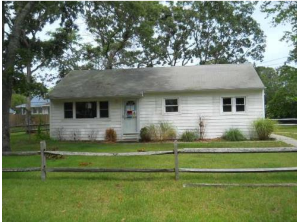
1 front elevation Date Taken: 7/21/2014 Taken By: Brook Benvenuti
