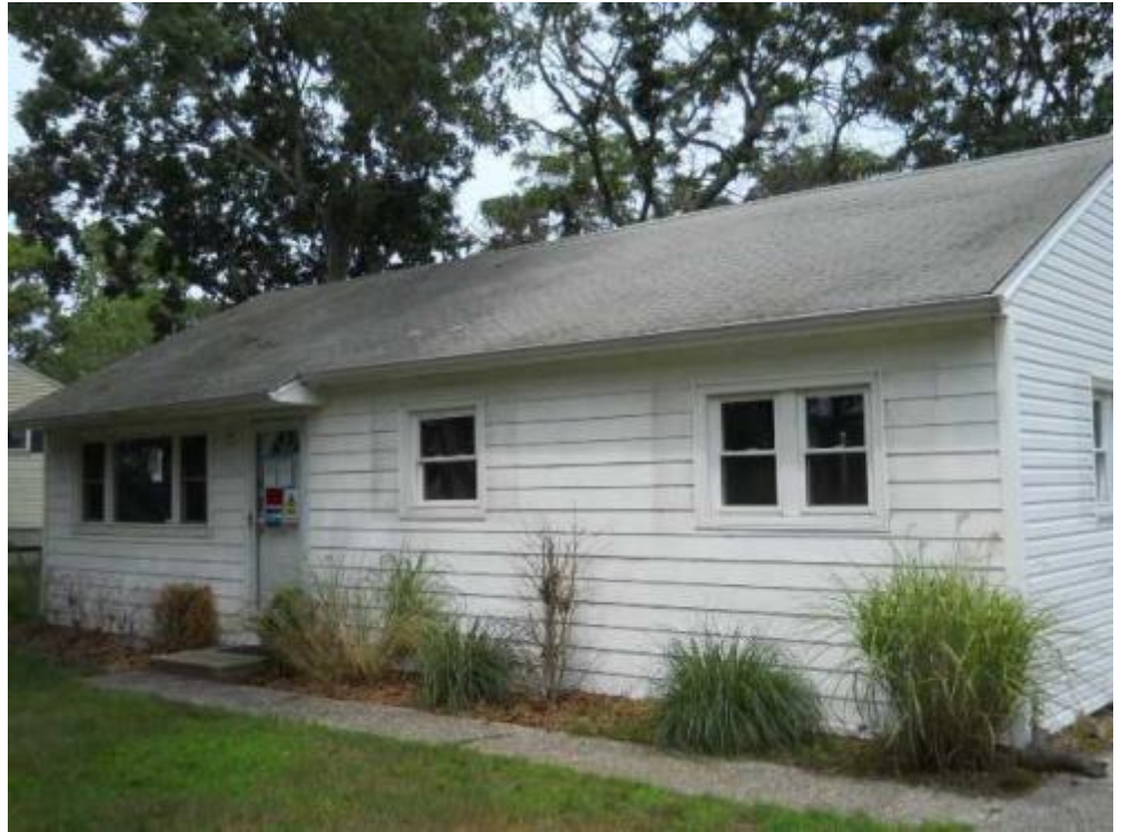
9 front elevation Date Taken: 7/21/2014 Taken By: Brook Benvenuti
