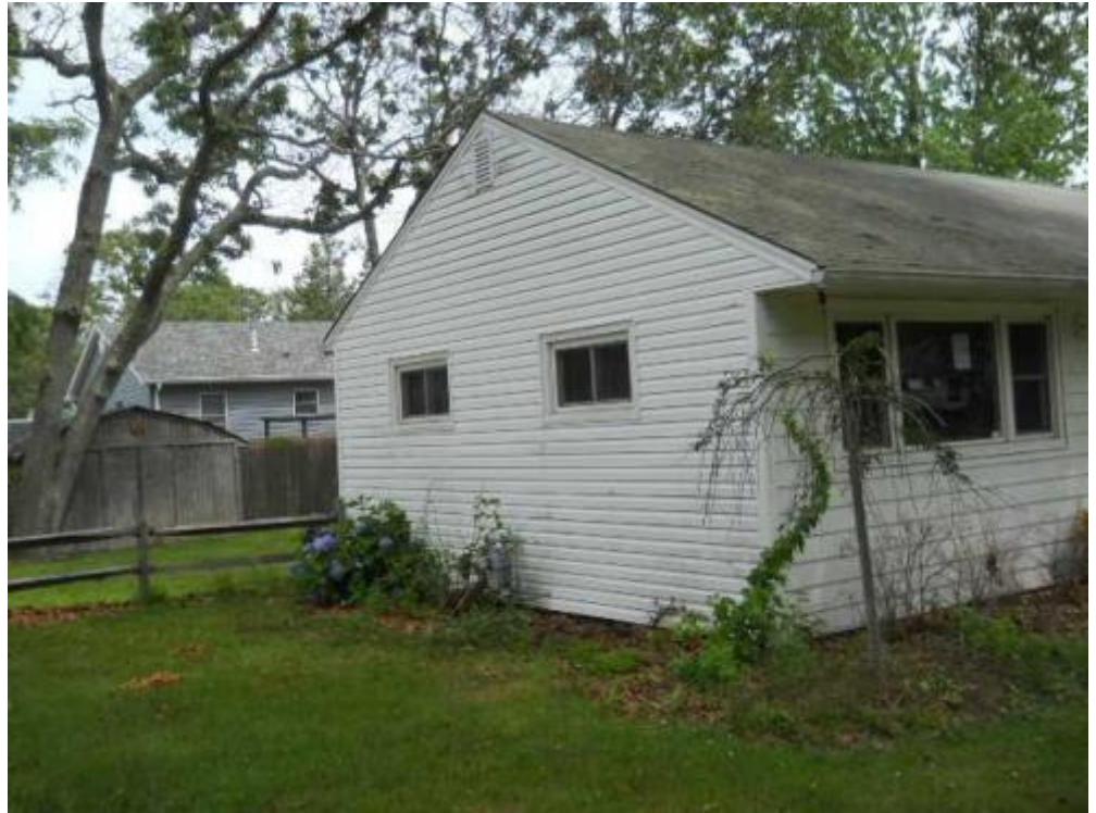
11 left elevation Date Taken: 7/21/2014 Taken By: Brook Benvenuti
