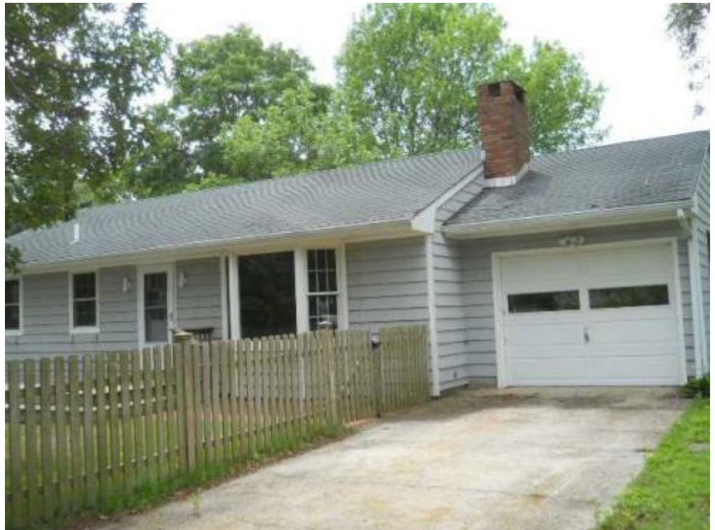
5 front elevation Date Taken: 7/21/2014 Taken By: Brook Benvenuti
