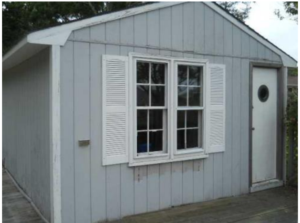
16 rear shed Date Taken: 7/21/2014 Taken By: Brook Benvenuti
