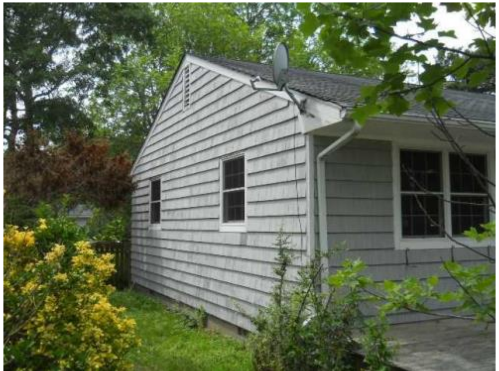
8 left elevation Date Taken: 7/21/2014 Taken By: Brook Benvenuti
