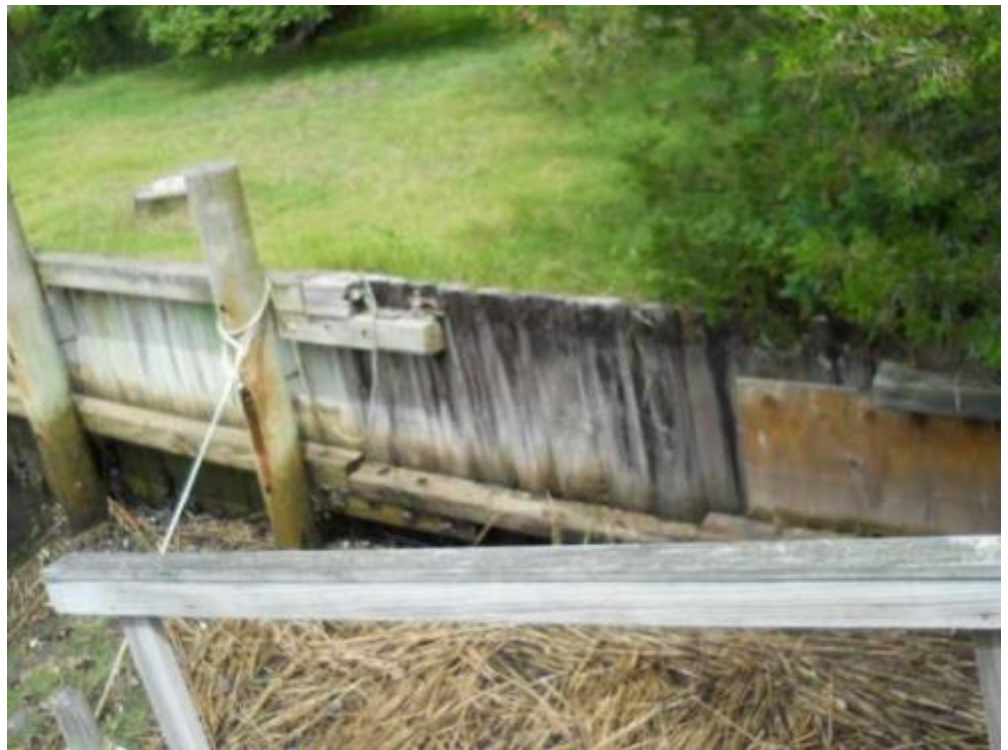
14 rear bulkhead Date Taken: 7/21/2014 Taken By: Brook Benvenuti
