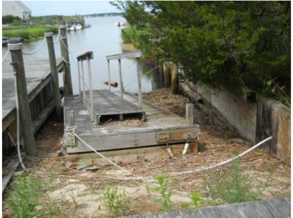
13 rear dock Date Taken: 7/21/2014 Taken By: Brook Benvenuti
