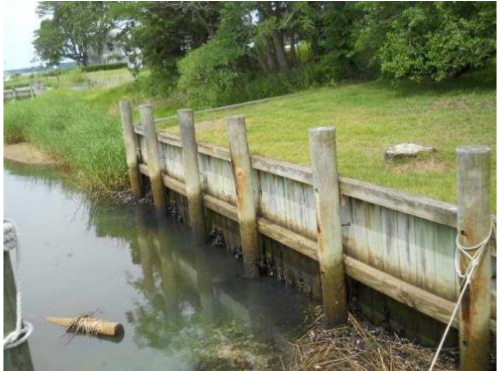
15 rear bulkhead Date Taken: 7/21/2014 Taken By: Brook Benvenuti
