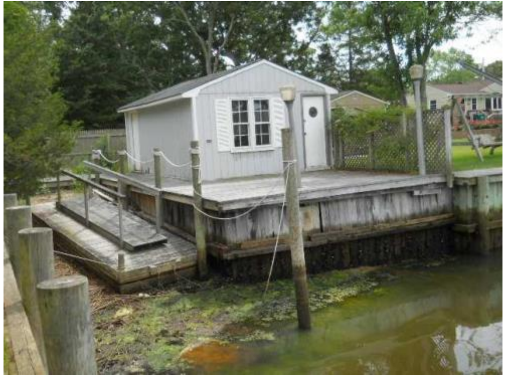
17 rear bulkhead Date Taken: 7/21/2014 Taken By: Brook Benvenuti
