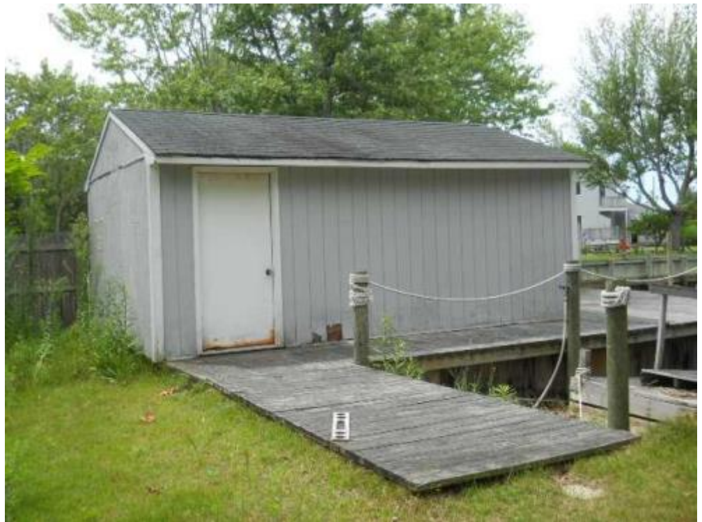
12 rear shed Date Taken: 7/21/2014 Taken By: Brook Benvenuti
