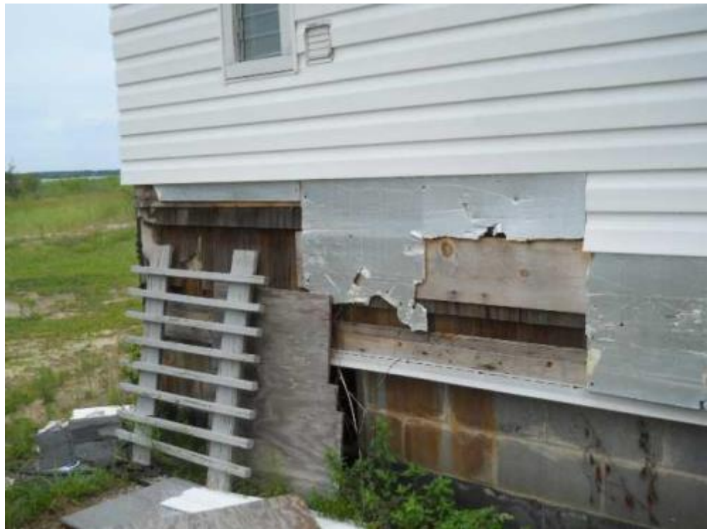
12 left elevation Date Taken: 7/21/2014 Taken By: Brook Benvenuti
