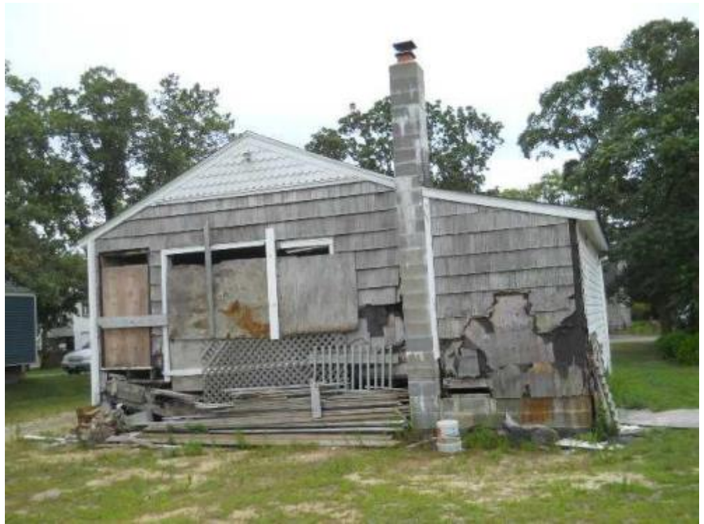
17 rear elevation Date Taken: 7/21/2014 Taken By: Brook Benvenuti
