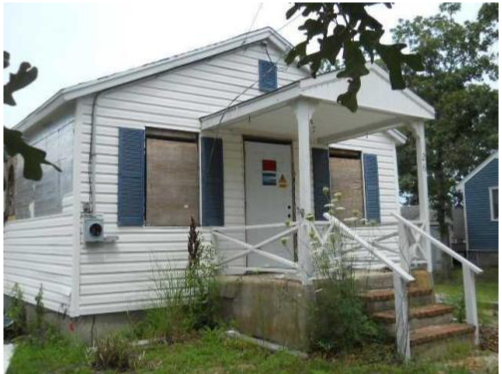
6 front elevation Date Taken: 7/21/2014 Taken By: Brook Benvenuti
