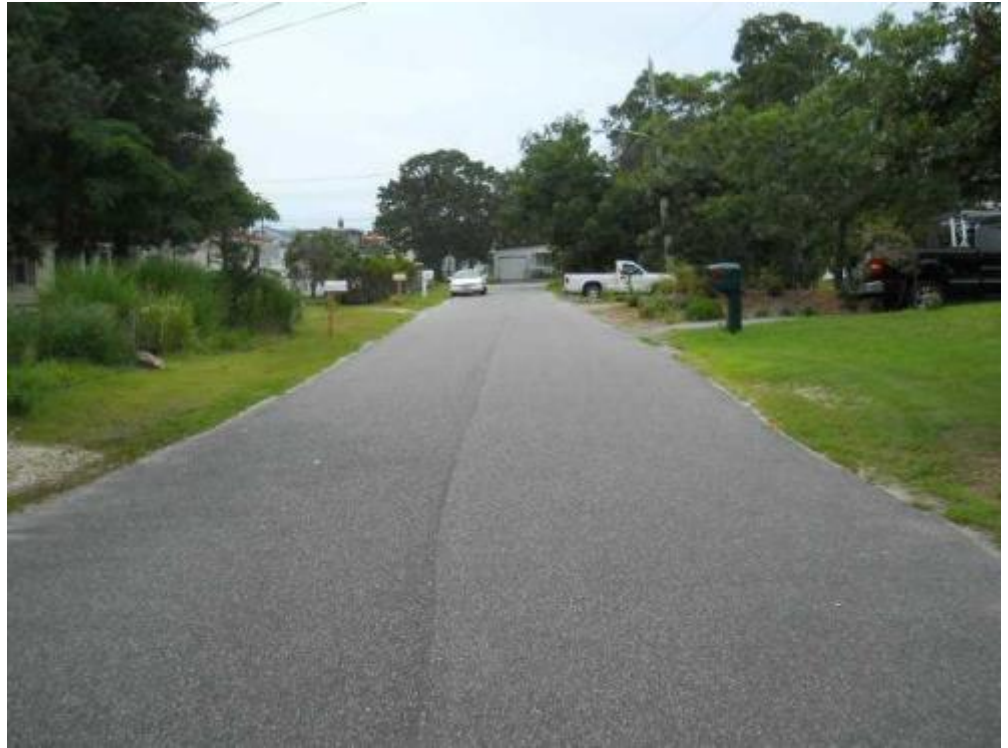
3 street left Date Taken: 7/21/2014 Taken By: Brook Benvenuti
