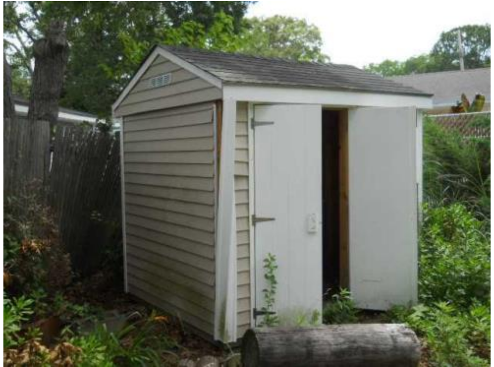
13 rear shed Date Taken: 7/21/2014 Taken By: Brook Benvenuti
