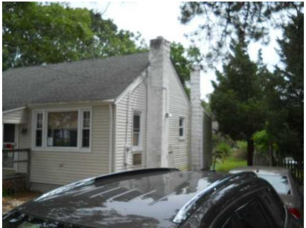
16 right elevation Date Taken: 7/21/2014 Taken By: Brook Benvenuti
