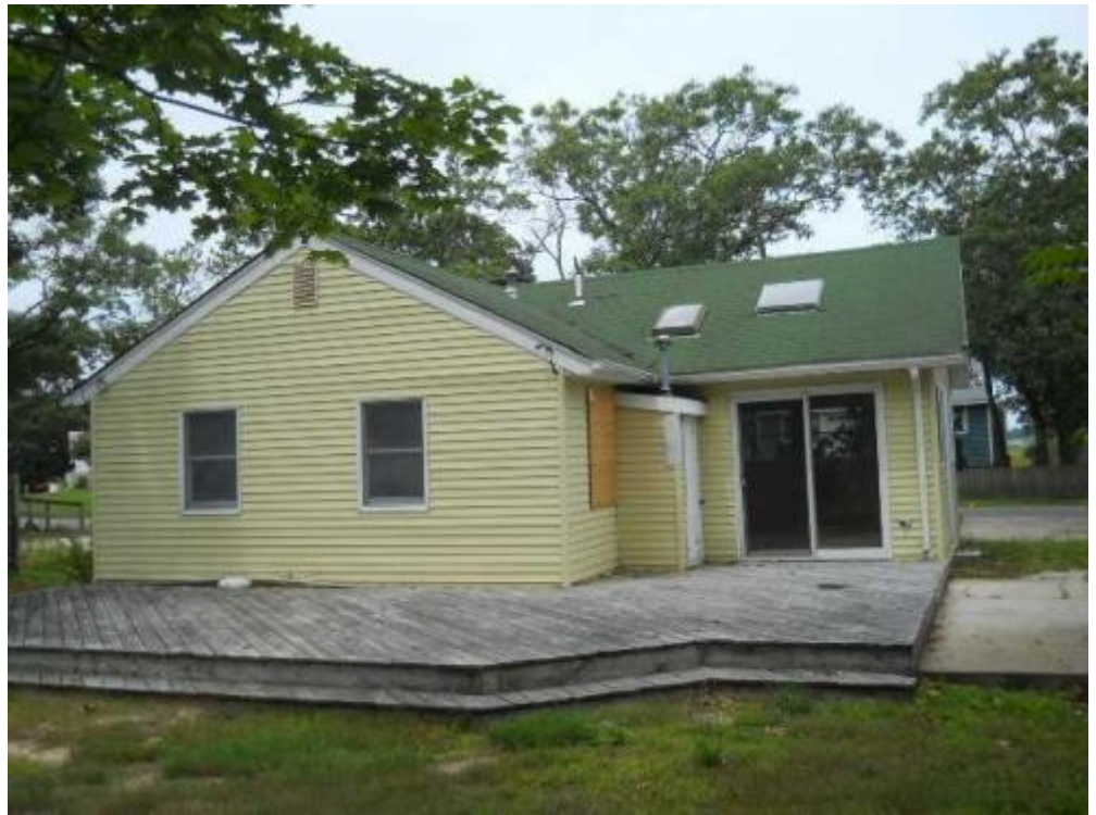
11 rear elevation Date Taken: 7/21/2014 Taken By: Brook Benvenuti
