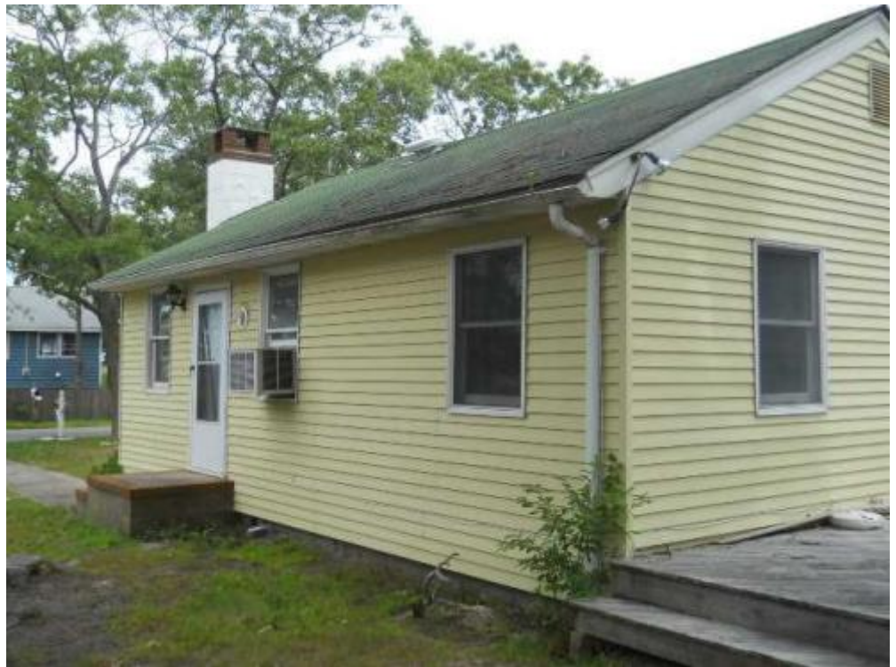
14 right elevation Date Taken: 7/21/2014 Taken By: Brook Benvenuti
