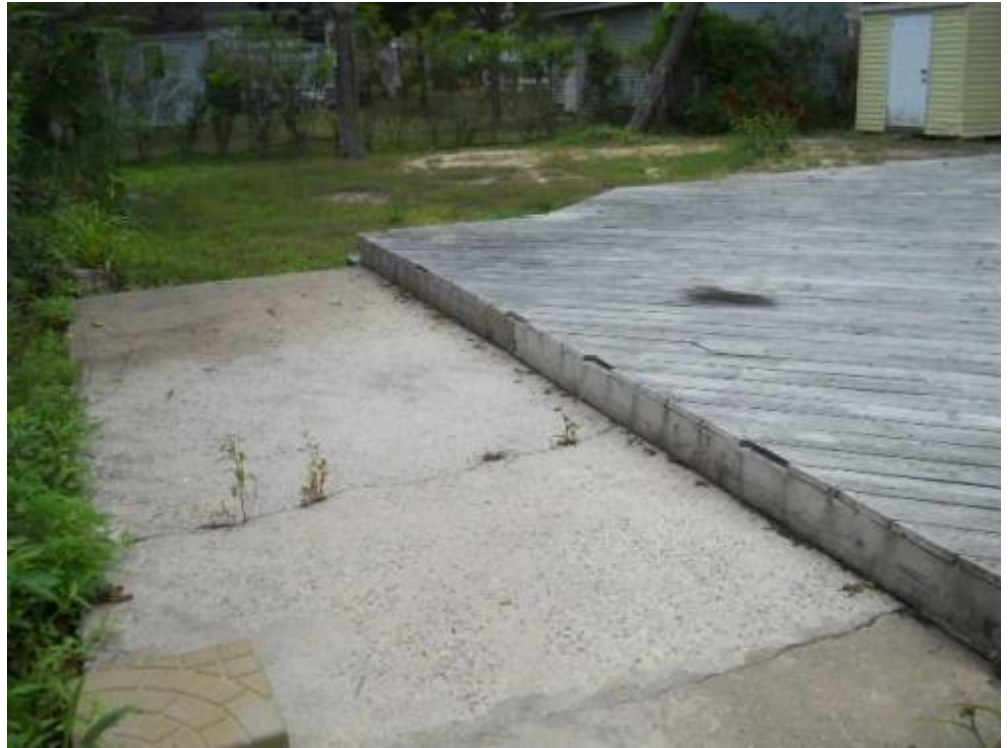
9 left concrete, deck Date Taken: 7/21/2014 Taken By: Brook Benvenuti
