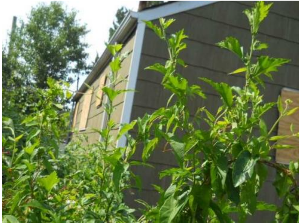
13 right elevation Date Taken: 7/20/2014 Taken By: Brook Benvenuti
