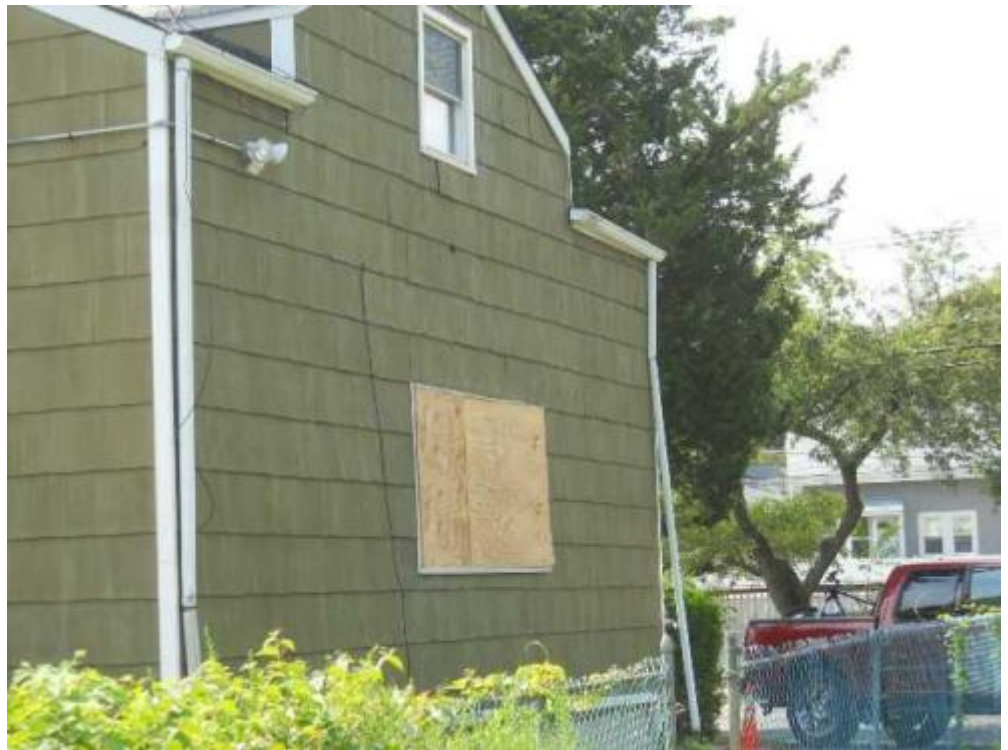
12 left elevation Date Taken: 7/20/2014 Taken By: Brook Benvenuti
