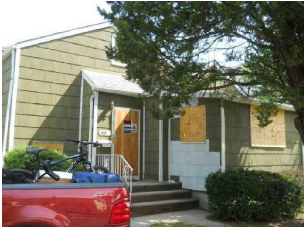
1 front elevation Date Taken: 7/20/2014 Taken By: Brook Benvenuti
