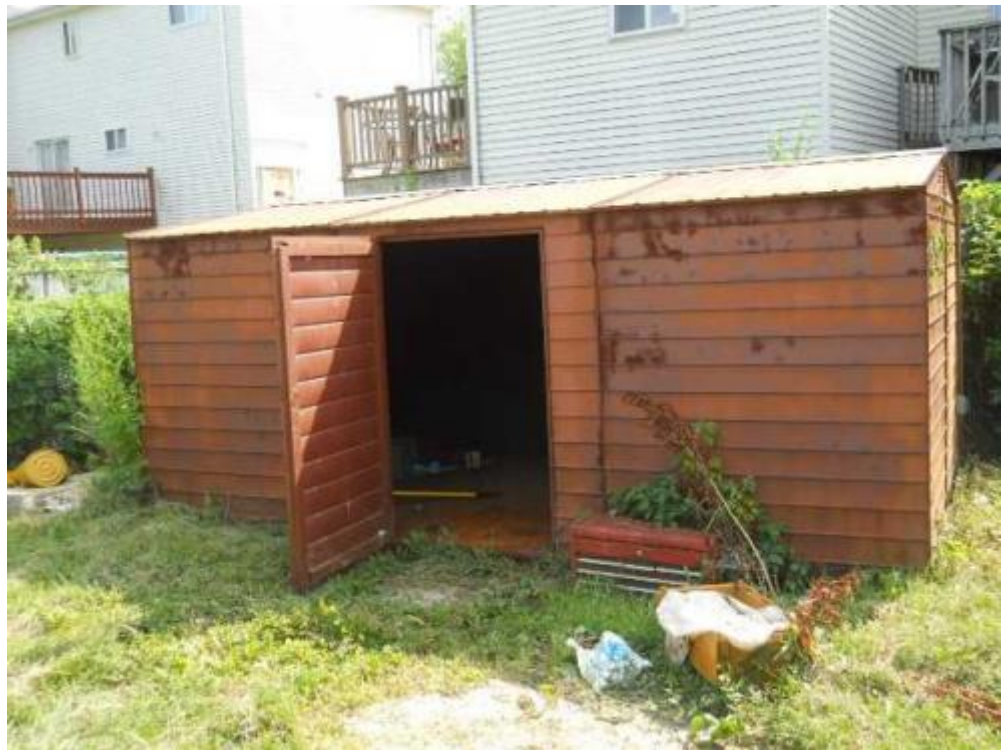
8 back yard Date Taken: 7/20/2014 Taken By: Brook Benvenuti detached structure
