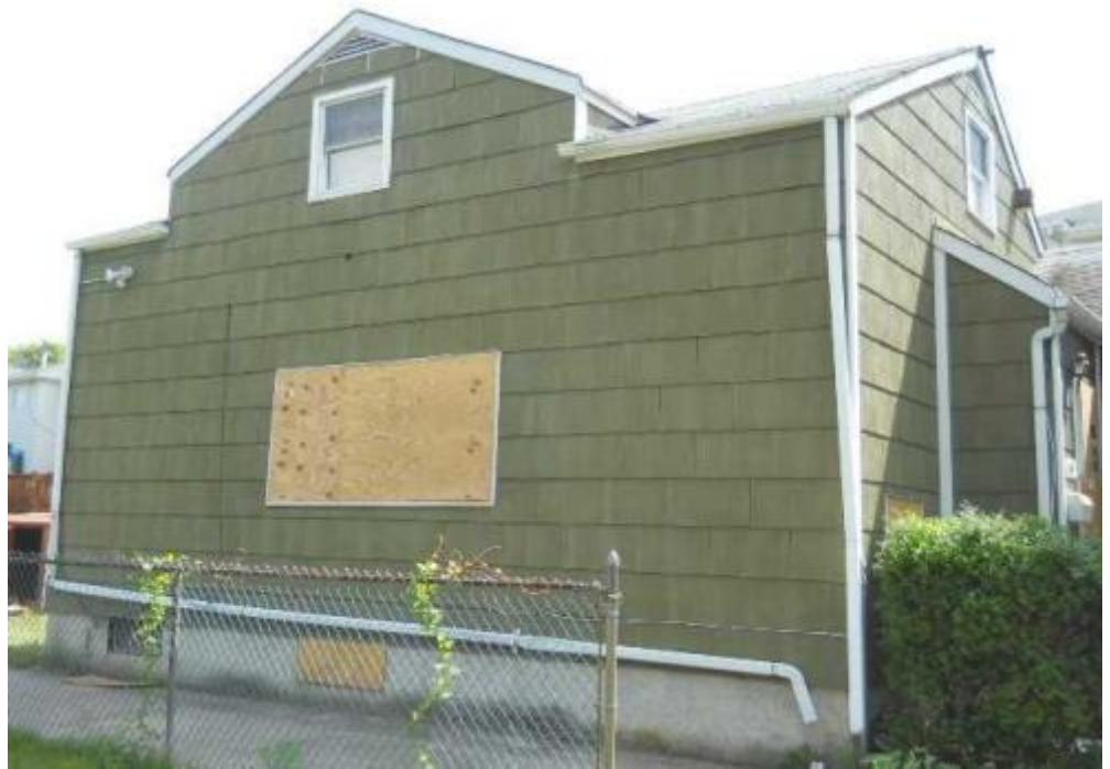
11 left elevation Date Taken: 7/20/2014 Taken By: Brook Benvenuti
