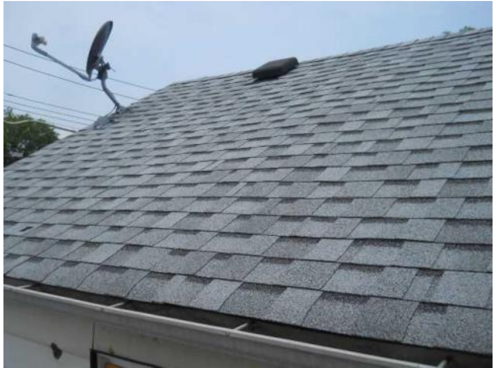
19 Roof Date Taken: 7/15/2014 Taken By: Brook Benvenuti
