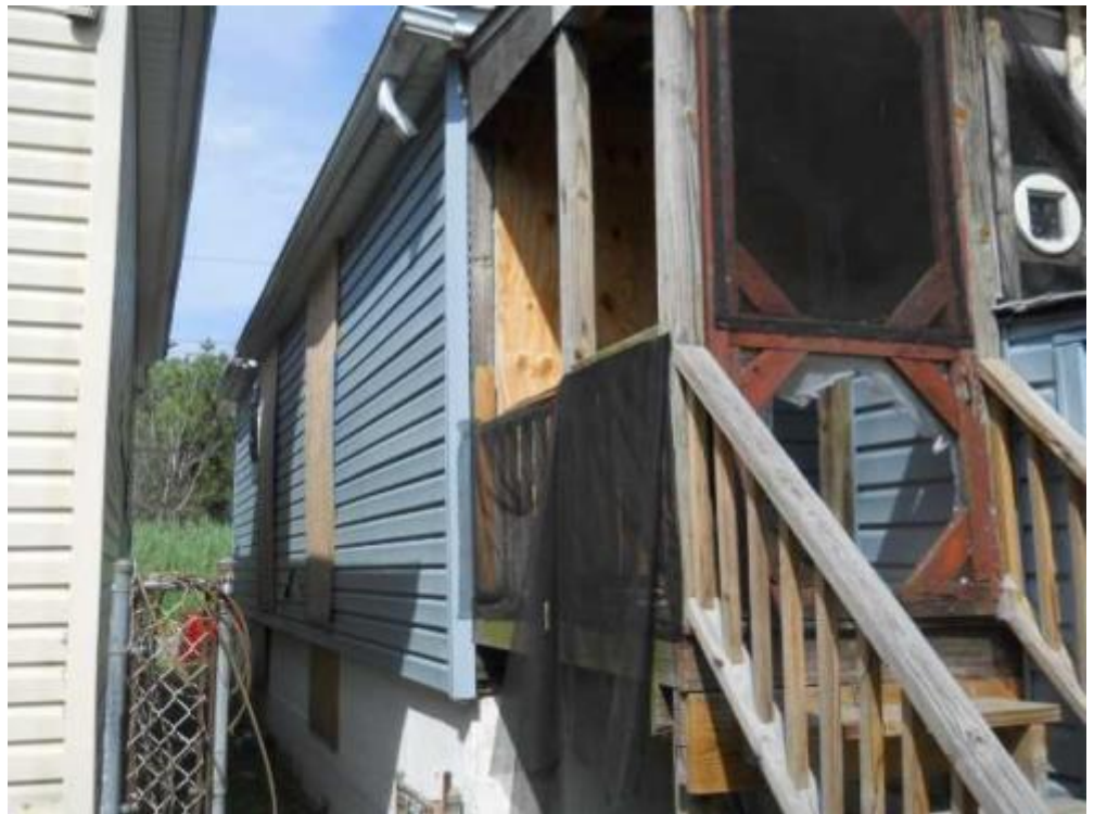
12 right elevation Date Taken: 7/19/2014 Taken By: Brook Benvenuti
