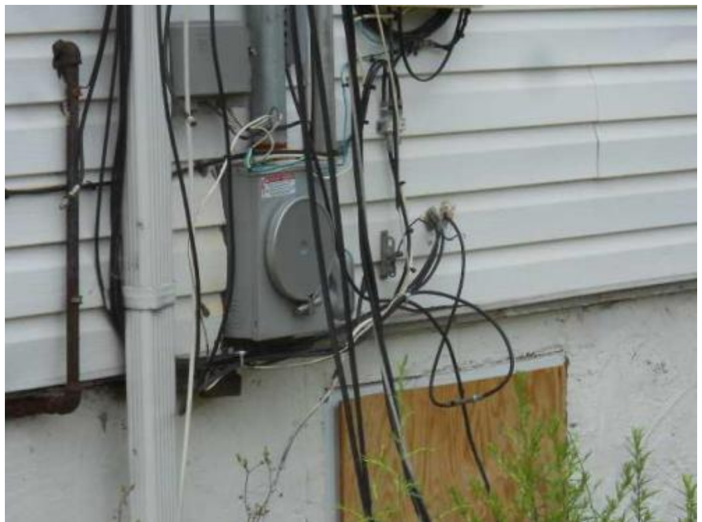
18 utilities off Date Taken: 7/16/2014 Taken By: Brook Benvenuti
