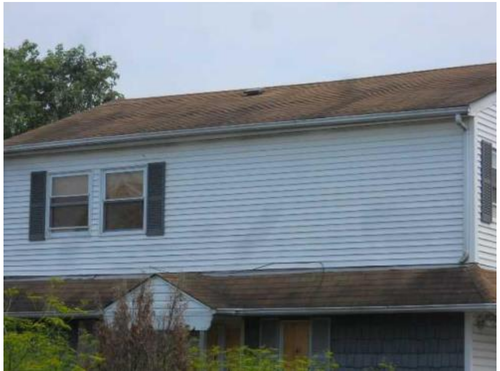
17 left roof Date Taken: 7/16/2014 Taken By: Brook Benvenuti
