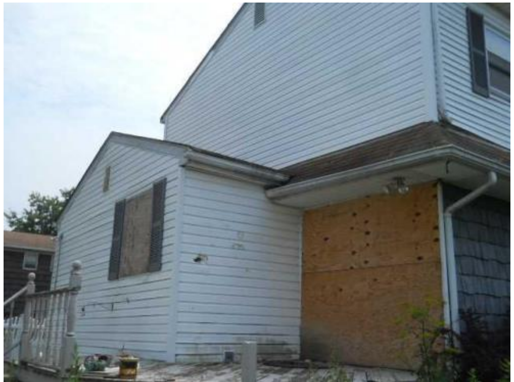
12 rear and deck Date Taken: 7/16/2014 Taken By: Brook Benvenuti
