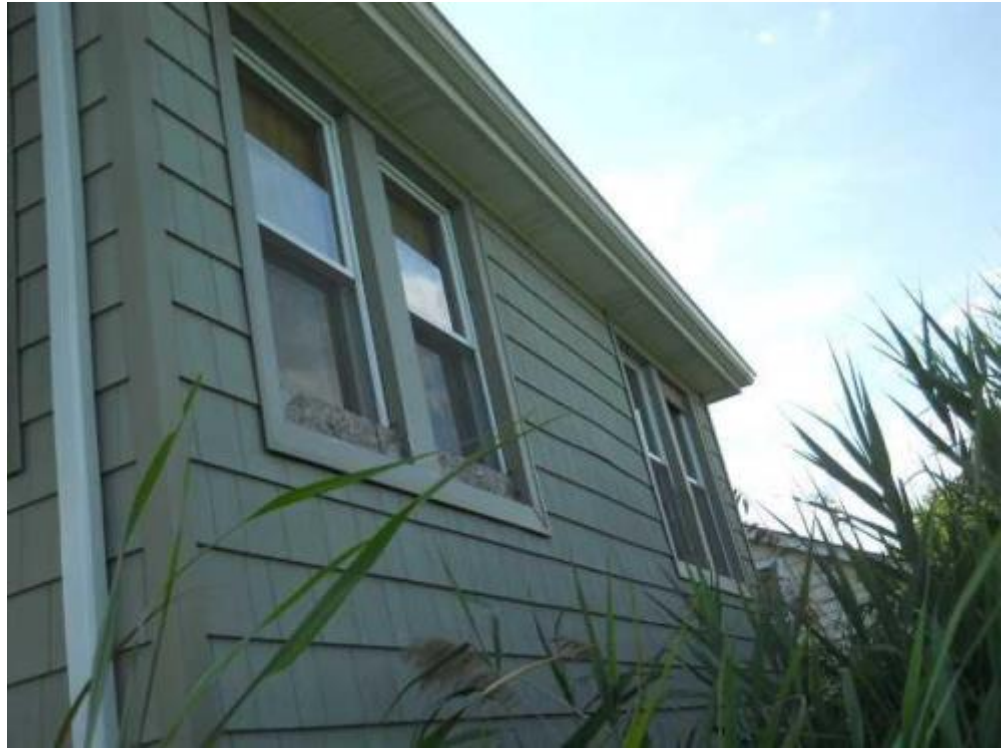
17 rear elevation Date Taken: 7/19/2014 Taken By: Brook Benvenuti
