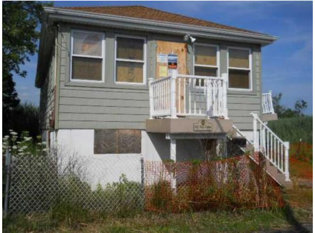
1 front elevation Date Taken: 7/19/2014 Taken By: Brook Benvenuti
