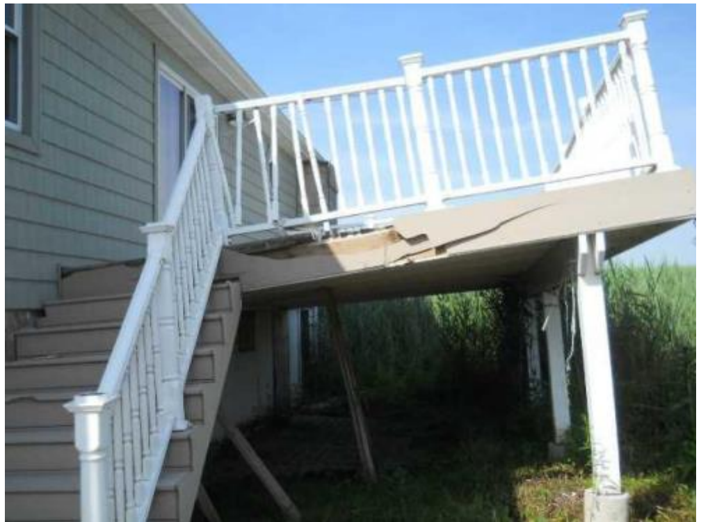
16 right elevation Date Taken: 7/19/2014 Taken By: Brook Benvenuti
