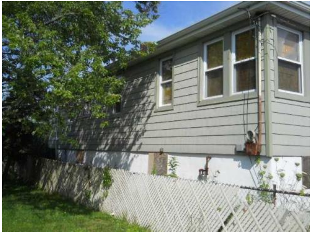
15 left elevation Date Taken: 7/19/2014 Taken By: Brook Benvenuti
