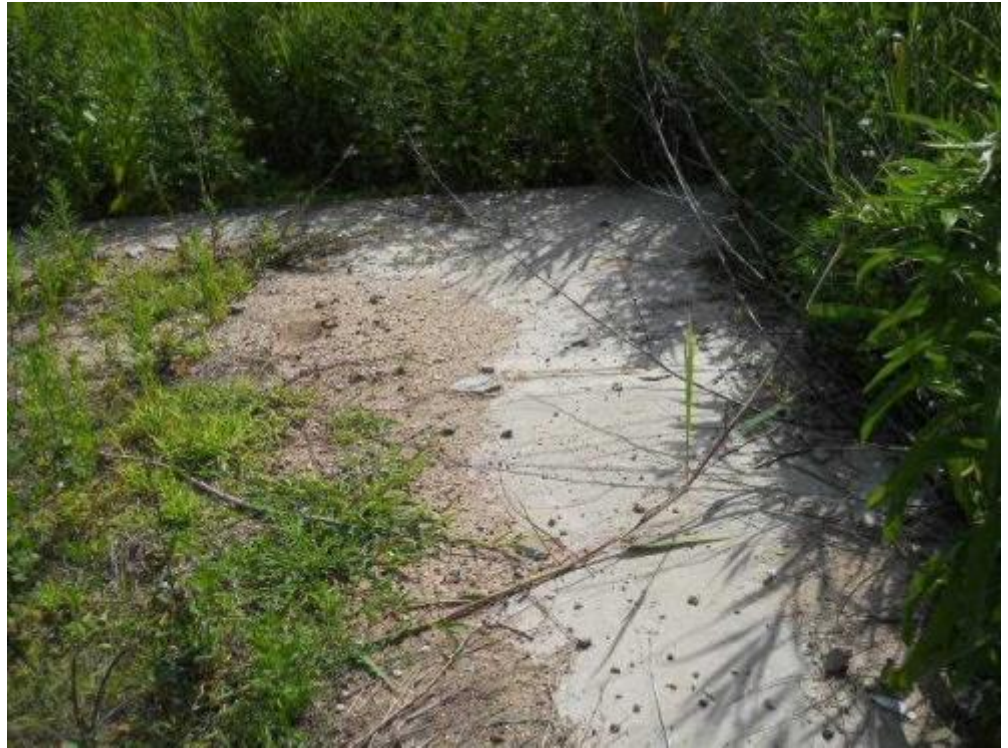
11 concrete slab Date Taken: 7/19/2014 Taken By: Brook Benvenuti
